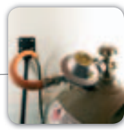
Gas regulator with over-pressure protection
